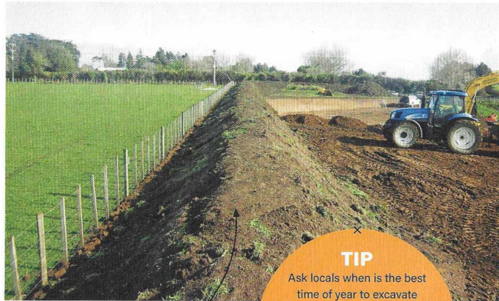
A 2m high berm was created along one boundary, using topsoil from the site, to create instant shelter. This is now covered in plants and trees.
